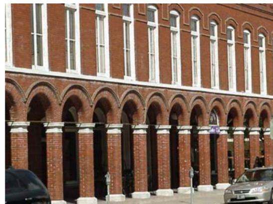
**Arcade:** A covered walk with a line of arches along one or both long sides, often with shops and offices along one side. Differentiated from a colonnade because it is a series of arches (usually heavy masonry) instead of columns. (*Variation: Colonnade, Gallery, Stoa*)
