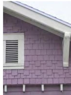
Random-width cut wood or fiber-cement shingles with mitered corners or 5/4 x 6-inch corner board trim
