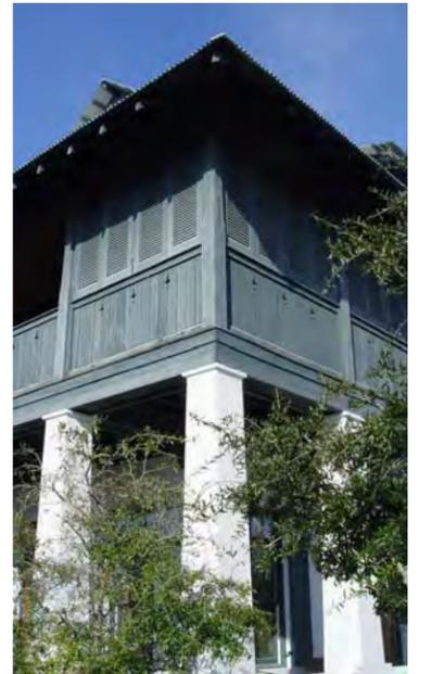
The upper floors have lighter wood construction and therefore have smaller sections and thinner profile wood columns or posts. More vernacular designs are most common with simple square sections of 4x4, 6x6 or 8x8. More refined designs have chamfered corners, tapered shafts and simplified capitals and bases. Turned wood columns with some elaboration are less common.
