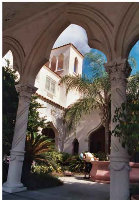
**Colonnade:** A number of columns arranged in order, at intervals called intercolumniation, supporting an entablature and usually one side of a roof. This element is differentiated from an *arcade* because it is a series of columns instead of arches. (Variation: **Arcade, Gallery, Loggia, Pergola, Porch, Portico, Stoa, Veranda**)
