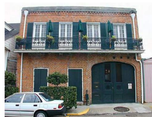
**Carriageway:** A wide *passage* along one side of a building, penetrating through the building underneath a habitable space above, connecting the street to the
